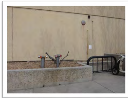
BMSB standpipe and wet pipe connections
