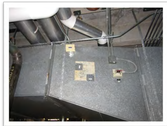
Typical abandoned relay and smoke detector
