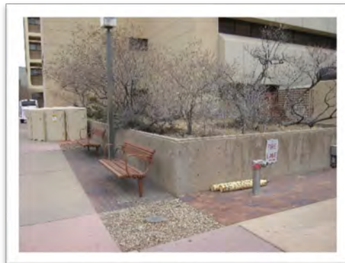
BRF wet pipe fire department connection
