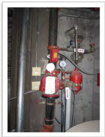
BRF main fire protection riser
